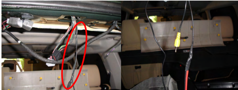
(this is the newly threaded cabling, gently pull most into the boot area – the power cable connection will eventually end up almost inside the rubber tube)
