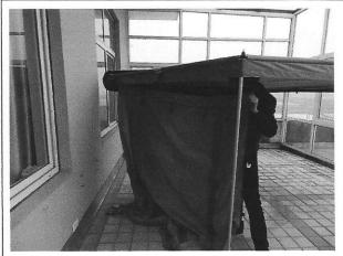
Slide the tent walls into the sail track at the bottom of the awning mounting plate.
