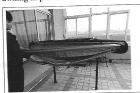
Unfold the awning slowly and stop in first triangle unfolded completely, meanwhile hold the other part of the awning.
