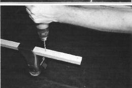
Drill at least 2 holes for each L-shaped bracket. We highly recommend to take the racks off your car for this prosedure.
