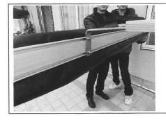
Fix the awning to the mounting brackets with M6 bolts.
