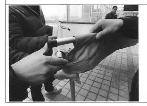
Slide the mosquito net into the sail track at the bottom of the awning mounting plate.
